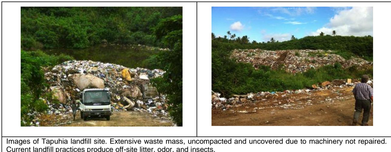
42. Following the construction of cell 2, the uncompacted, uncovered waste in cell 1 can then be compacted and covered. This allows the construction of an access road on cell 1 waste for plant and equipment to install quarry wall protection (liner and clay cover) for a second lift in cell 1. Once the second lift is completed, further secure landfilling capacity will be available in this cell.
